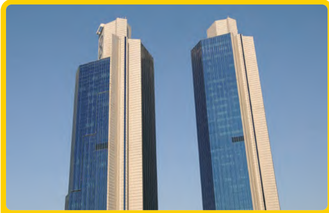
Sabancı Center – İstanbul, 1991
